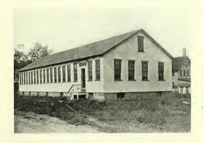
first floor is used for manufacturing purposes, the stock room being in the basement. It is equipped with hydraulic elevator. The power is furnished by a gas engine.
